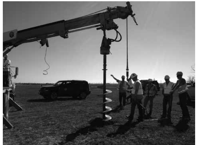
Setting of the new CBL station. Digging a 2 foot diameter hole 6 feet deep. CDOT Region 1 provided the equipment to drill four holes for the new CBL. From left to right: J. Faust (on the drill rig), E. Mundt, CDOT; T. Meeks, JFSato; D. Kuxhausen, T. Perazzo, C. Raml, Woolpert; K. Kucharczyk, JFSato
