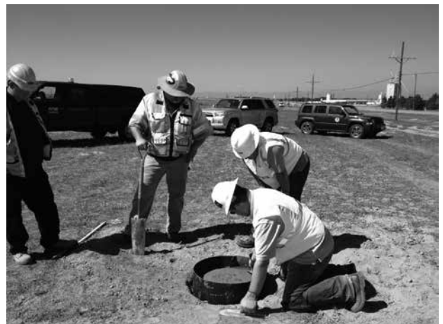
Setting of the new CBL station. A geodetic mark is placed on top of the concrete. The concrete was provided by the Central Chapter of the Professional Land Surveyors of Colorado. The distances on the marks will be measured next year and the new CBL published at that time. The Denver skyline is visible in the background. From left to right: B. White, T. Bridgeman, CDOT; D. Kuxhausen, C. Raml, Woolpert
