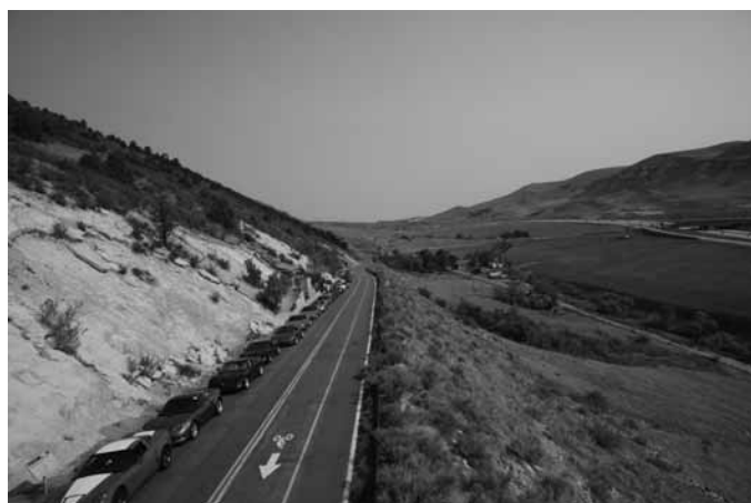
Figure 1. General view of the site, illustrating the photos taken up and down the road for control purposes.
