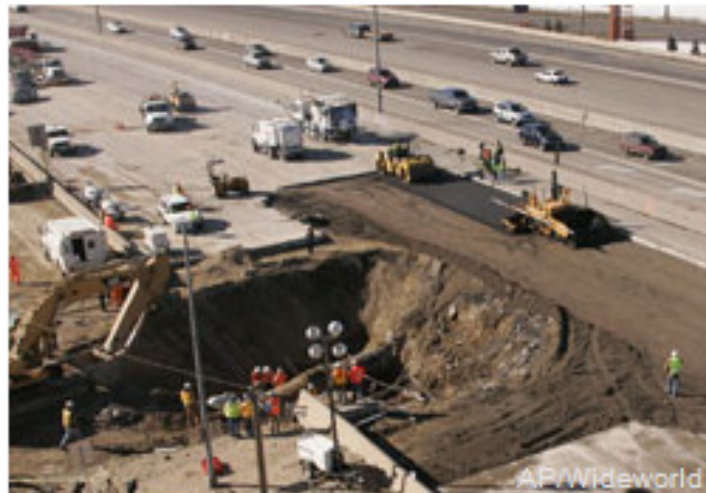
On Feb. 8, Denver Water employees remove aging, damaged pipe section that broke the day before. Massive sinkhole buckled a large segment of I-25.
