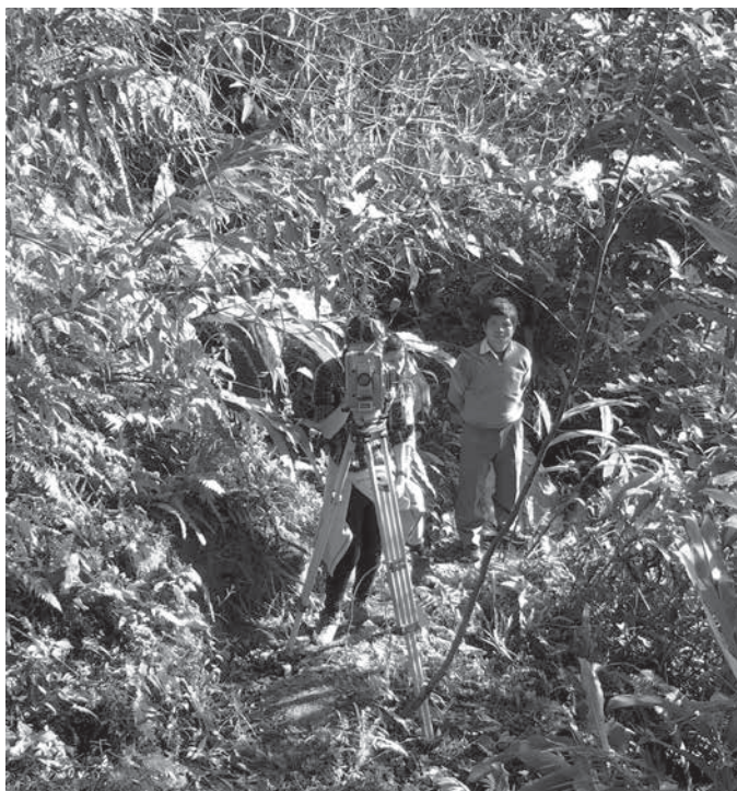
Travel team member Priscilla Dao uses a total station to survey a plot of land where a tank to serve the Godak school will be built. Photo Credit: Bryan Melonis, EWB Student
